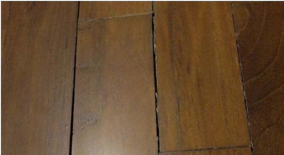
DEFECTS: Cracks in parquet floor. PHOTO COURTESY OF CELINE CHENG
